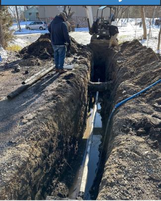
The sewer pipes were replaced at the caretaker house and a section at the clubroom. Also, The tree in the middle of the parking lot was removed.
